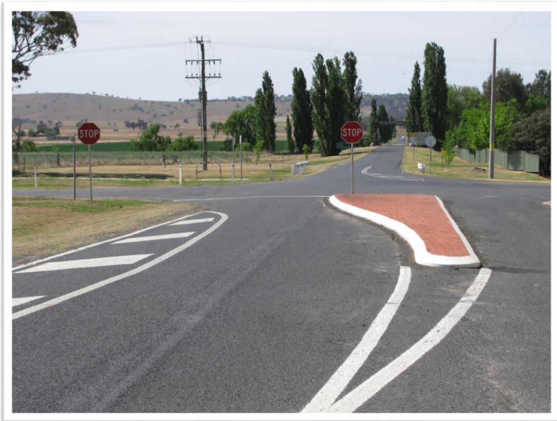
Intersection treatment Campbell Street Coolah which has changed the location of Give Way signs
